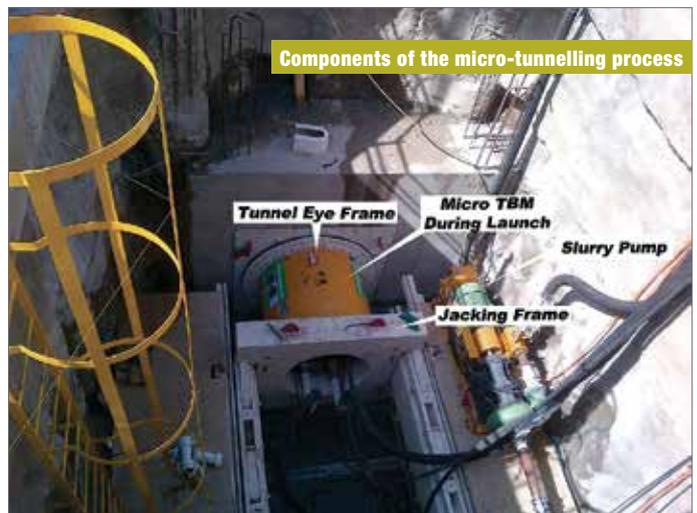
Components of the micro-tunnelling process
