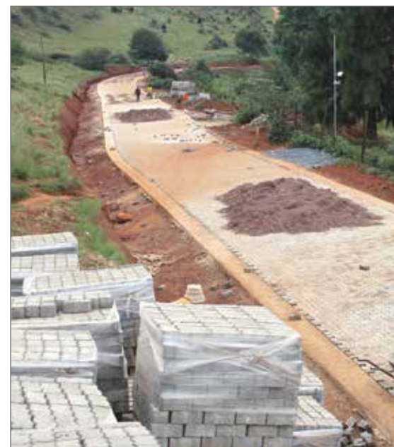
Working on edge restraints, screeding and paving
