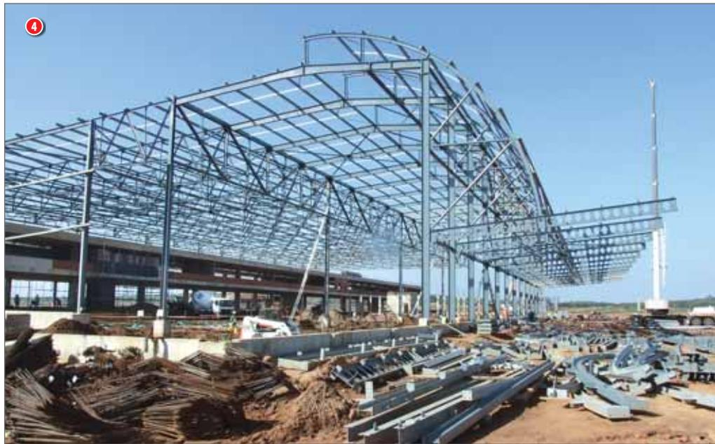
main girders being tied into the upper plant room level as continuous elements. All in-service longitudinal movement was then controlled by sliding teflon pad bearings at the peripheral support points.
