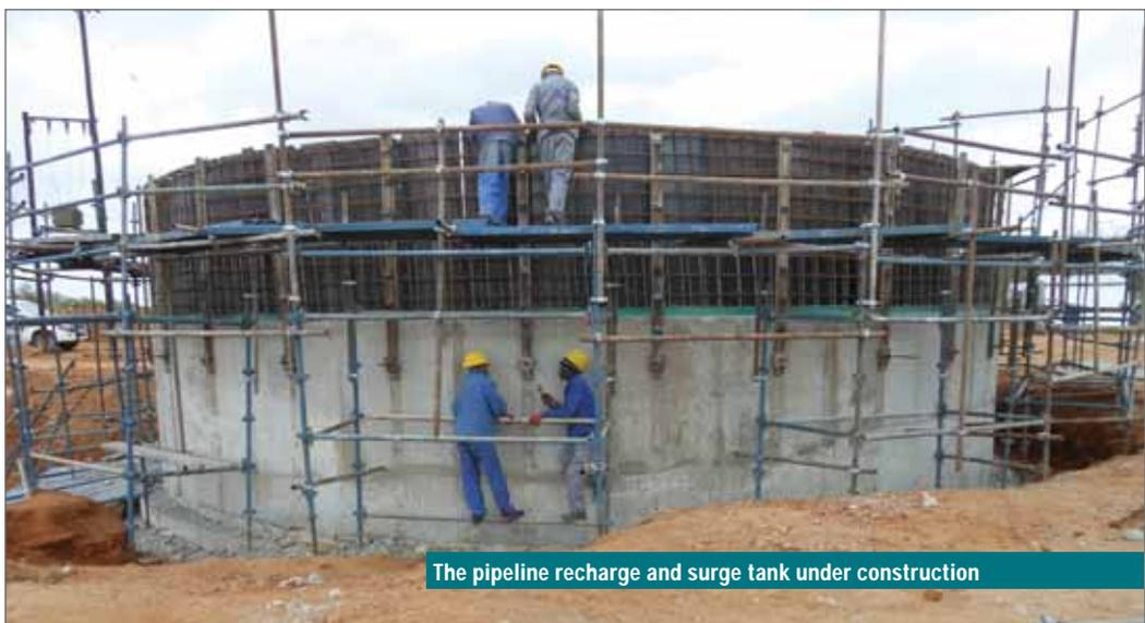
The pipeline recharge and surge tank under construction
