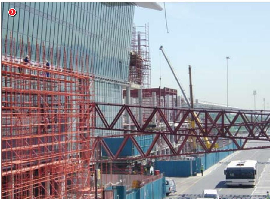
5 General view of the construction of the structural steel domestic departures lounge and arrival corridor over the existing airside road with the central terminal building in the background. The building is supported on the concrete columns in the foreground which allow free access for the vehicles below the building
