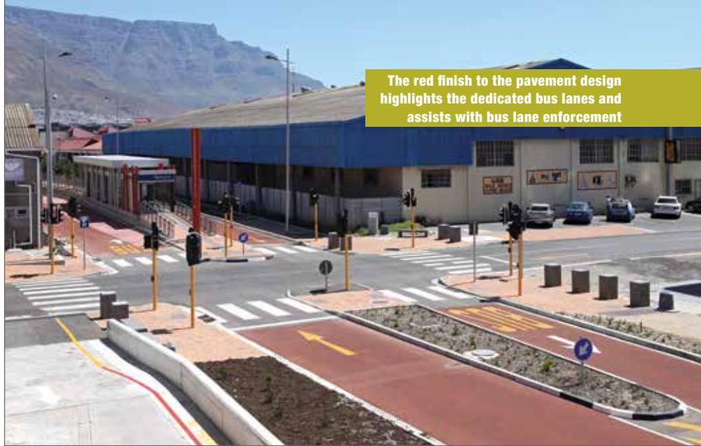
The red finish to the pavement design highlights the dedicated bus lanes and assists with bus lane enforcement
