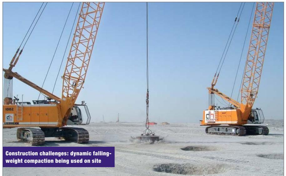
Construction challenges: dynamic falling-weight compaction being used on site
